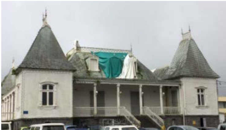
Figure 6 Tarpaulins Laid to Prevent Ingress of Rainwater
