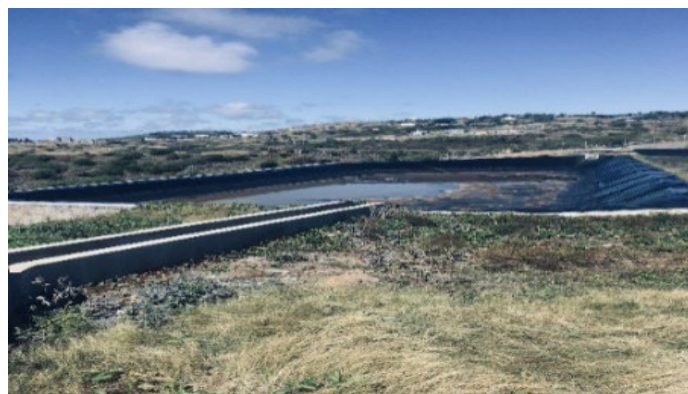
Figure 14: No water retained in the pond at Roche Bon Dieu for Anse Ally site
