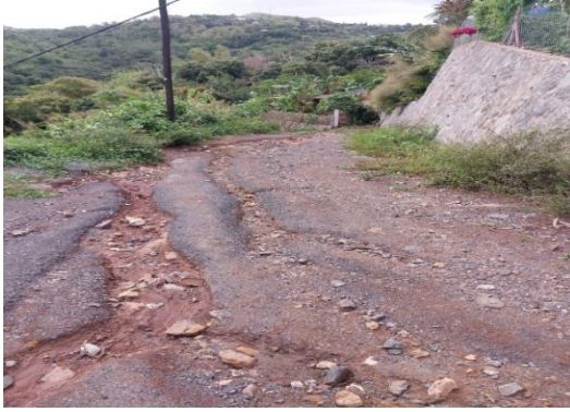
Figure 6 - Natural drains along access road near retaining wall at Pavé La Bonte
