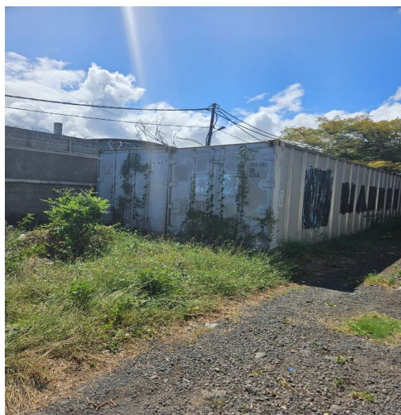
Figure 2 – Containers used as Stores in the compound of CSD at Plaine Lauzun
