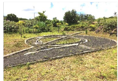
Illegal construction of health track on ASL leased for food crop production at Wooton
