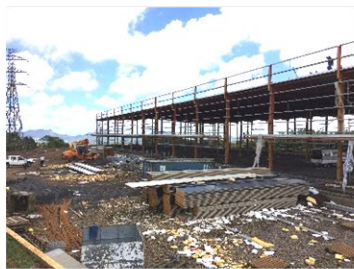
Agro-processing plant under construction on leased land at Wooton
