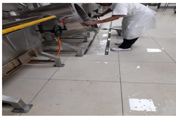
Fig 16 Food Hygiene and Safety: No proper drainage system-hot water spilling on the floor at SAJH
